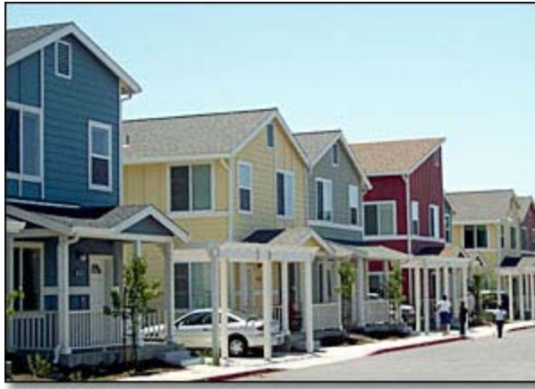
Edes Avenue Phase A in Oakland, a Habitat East Bay project creating 26 affordable houses for first-time homeowners"
