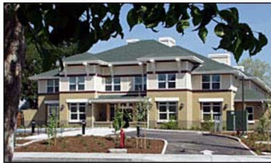
Fuller Gardens in San Leandro, supportive housing for residents with developmental disabilities
