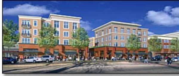
Multi-family condominium units in Richmond, CA
