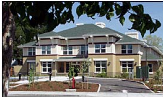
Fuller Gardens in San Leandro, supportive housing for residents with developmental disabilities
